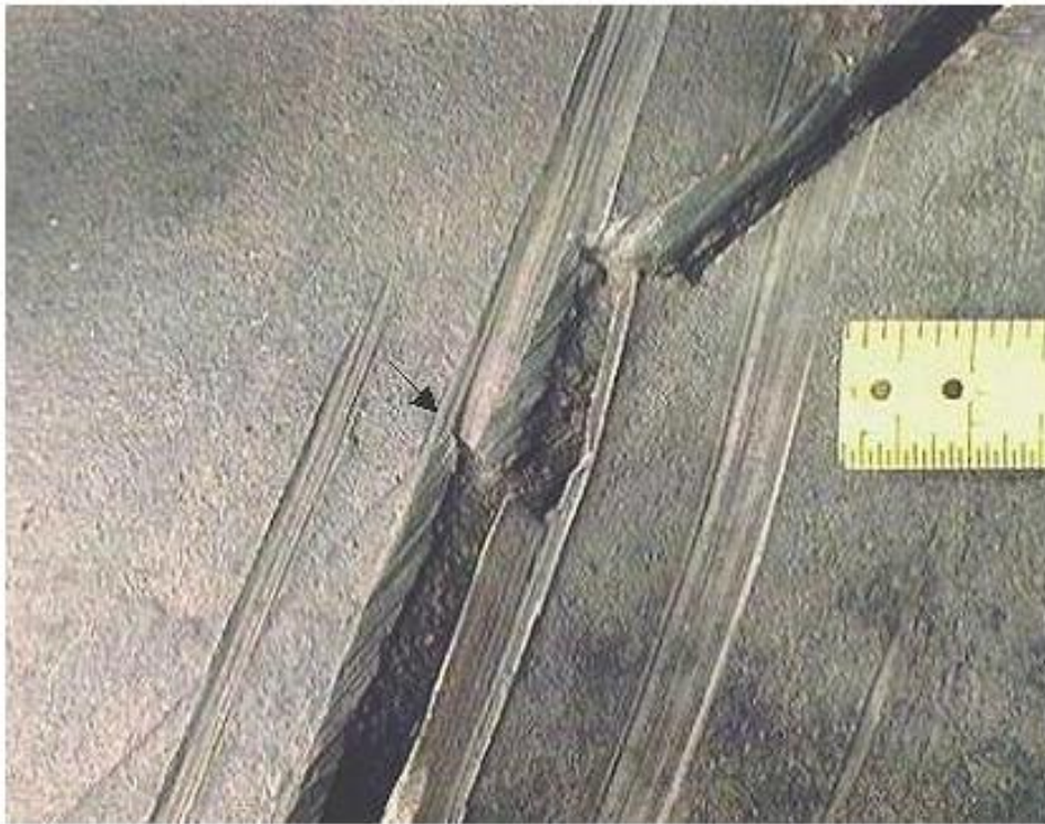
Figure 4-13 – Close-up photograph showing the gouges and the fracture origin (arrow) in one of the gouges.
