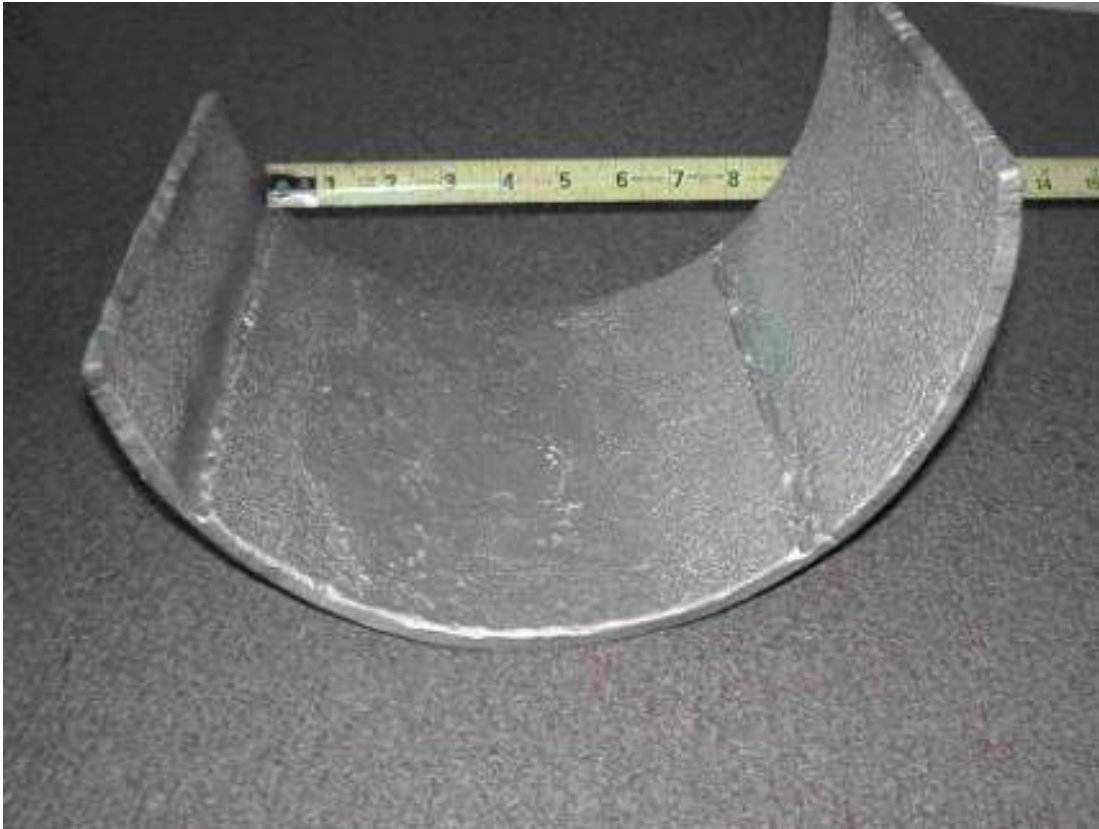
Figure 5-23 – Grooving corrosion in the carbon steel vapor line from an alkaline water wash drum in a sulfuric acid alkylation unit.
