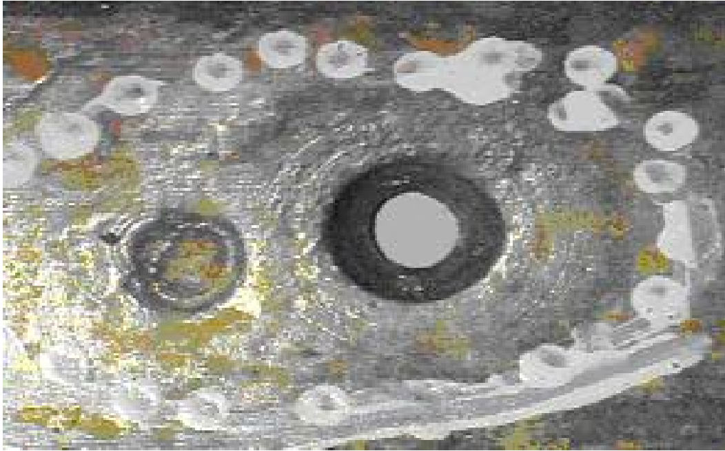
Figure 4-91 – Same pipe as Figure 4-90. Note the halo effect.
