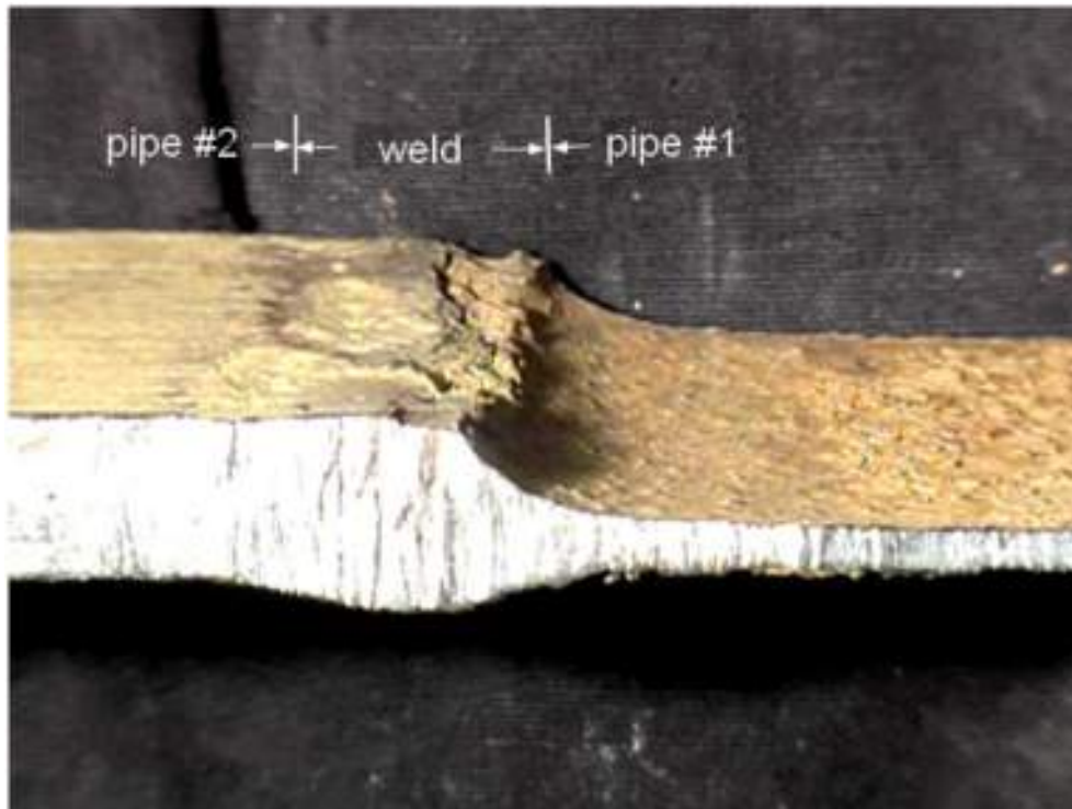
Figure 5-12 – Cross-section of a carbon steel pipe showing preferential corrosion of the pipe with high residual element content on the right, as compared to the low residual pipe section to the left of the weld (Reference 3).
