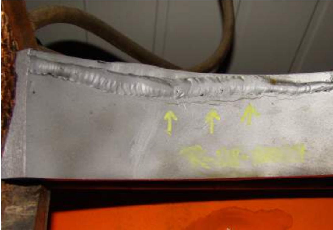
Figure 5-46 – Overhead interstage knockout drum vapor outlet nozzle.
