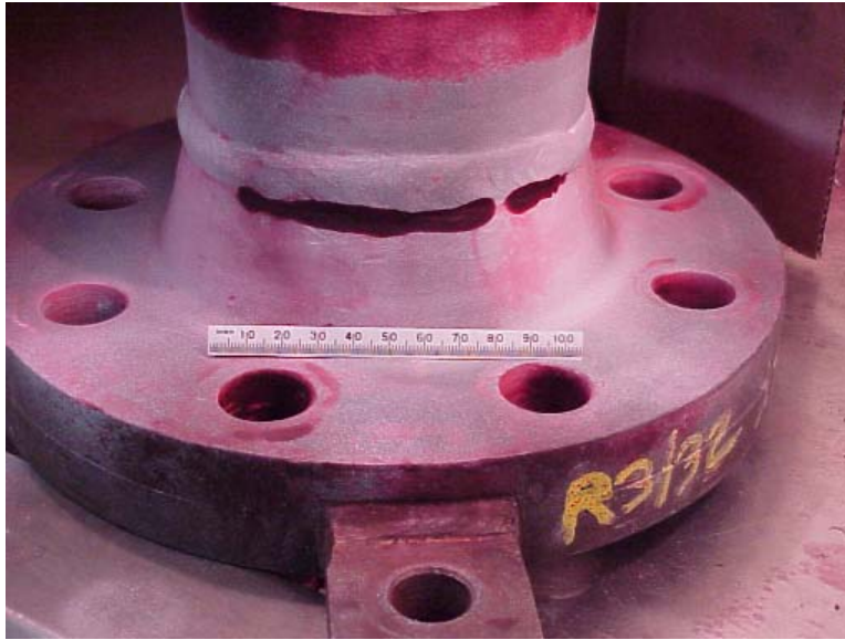
Figure 4-41 – Failure of nickel alloy DMW joining HP40 (Nb modified) tube to 1.25Cr-0.5Mo flange in a Steam Methane Reformer due to cold hydrogen disbonding of the buttering layer. Process temperature 914°-941°F (490° to 505°C), Pressure (2.14 Mpa), H 2 content 10-20% (off-gas).
