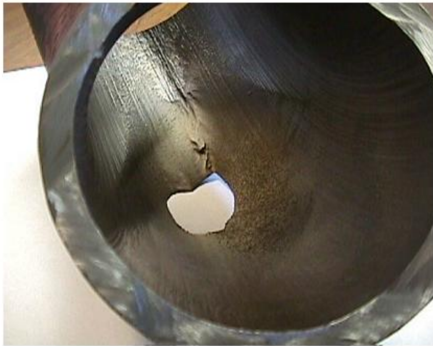
Figure 4-44 – Erosion of a 9Cr-1Mo coker heater return bend.
