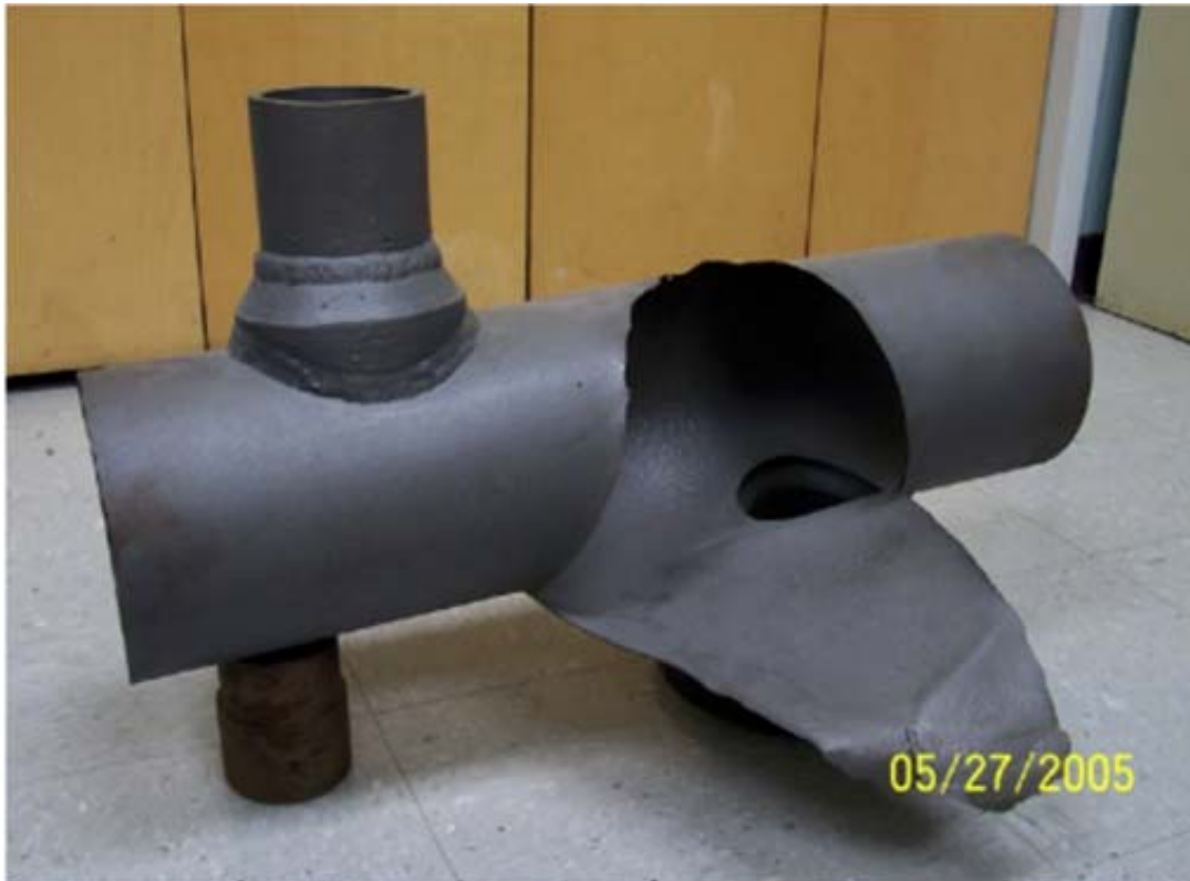
Figure 4-116 – Sulfidation failure of NPS 8 carbon steel pipe. Note the relatively uniform thinning that resulted in a sizeable rupture.
