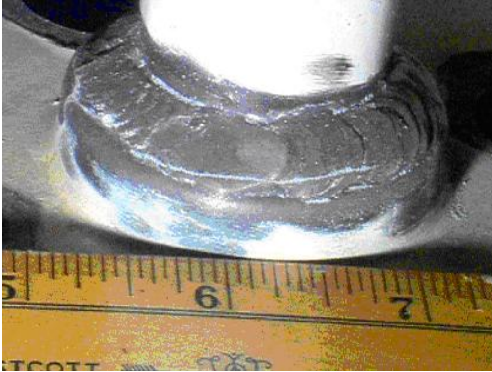
Figure 4-57 – Vibration induced fatigue of a 1-inch socket weld flange in a thermal relief system shortly after startup.
